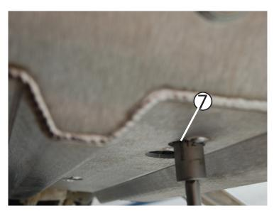
Using a 12mm socket, tighten the (4) nuts down on the underside of the plate. No thread locker is necessary here since these are locking-type nuts.
